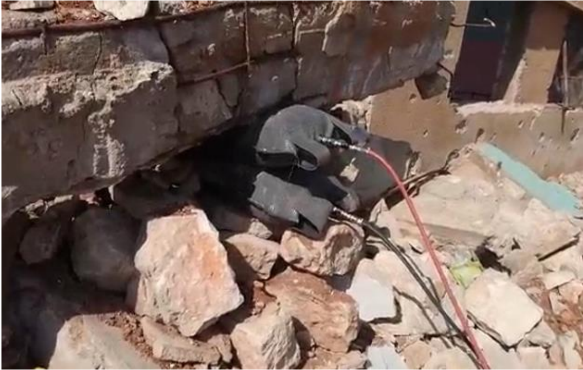
Photos of previous work: Locally made lifting airbags raising tons of rubble (above) and placement of insulation made locally with recycled plastic (below).
